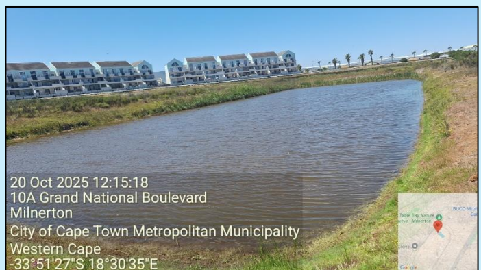
Figure 8: Fixed-point photograph of the Dam, taken on 20th of October 2025.
