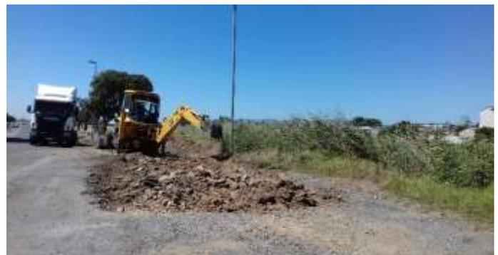
Figure 58. Breaking up the compacted infilling.
