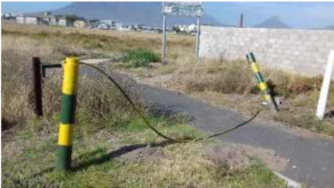
Figure 62. Destroyed access control cable.
