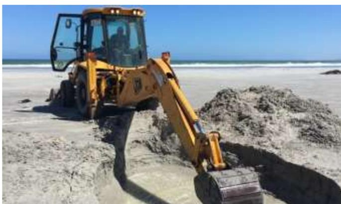
Figure 38. Excavator starting to cut the trench.
