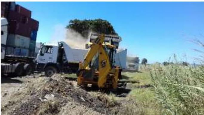
Figure 59. Removing the gravel material out of the wetland.
