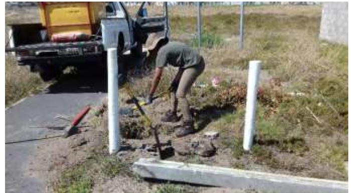
Figure 63. Field team repairing access control cable.
