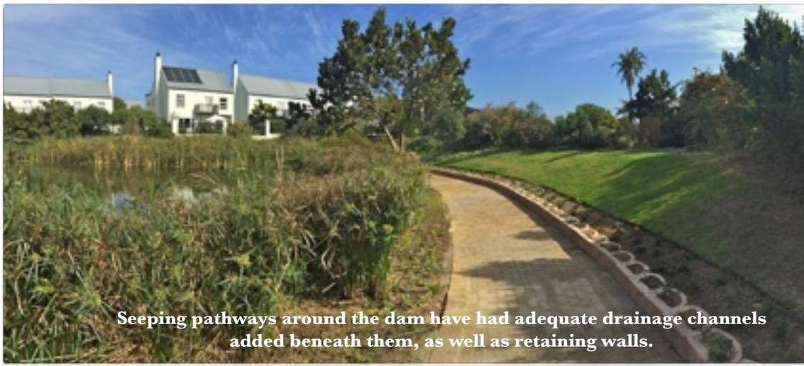
Seeping pathways around the dam have had adequate drainage channels added beneath them, as well as retaining walls.
