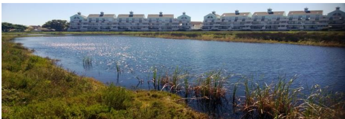
Figure 10: Fixed point photography of the Dam, taken on 12 September 2014.
