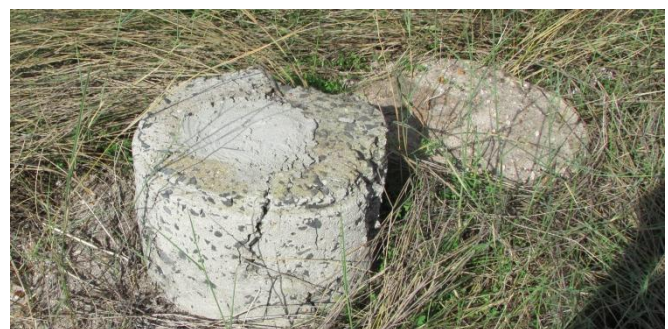
Figure 2: One of the old boreholes which is now closed.
